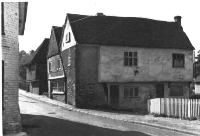
B. The range of buildings B and C prior to demolition.
