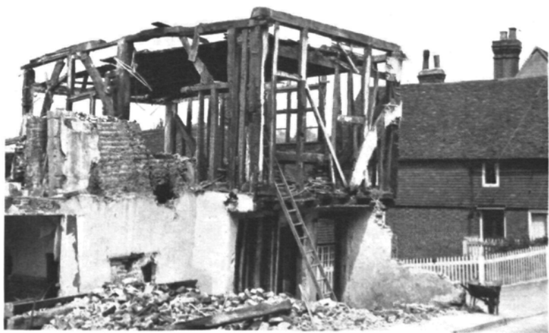
B. The solar wing of C in course of demolition.
